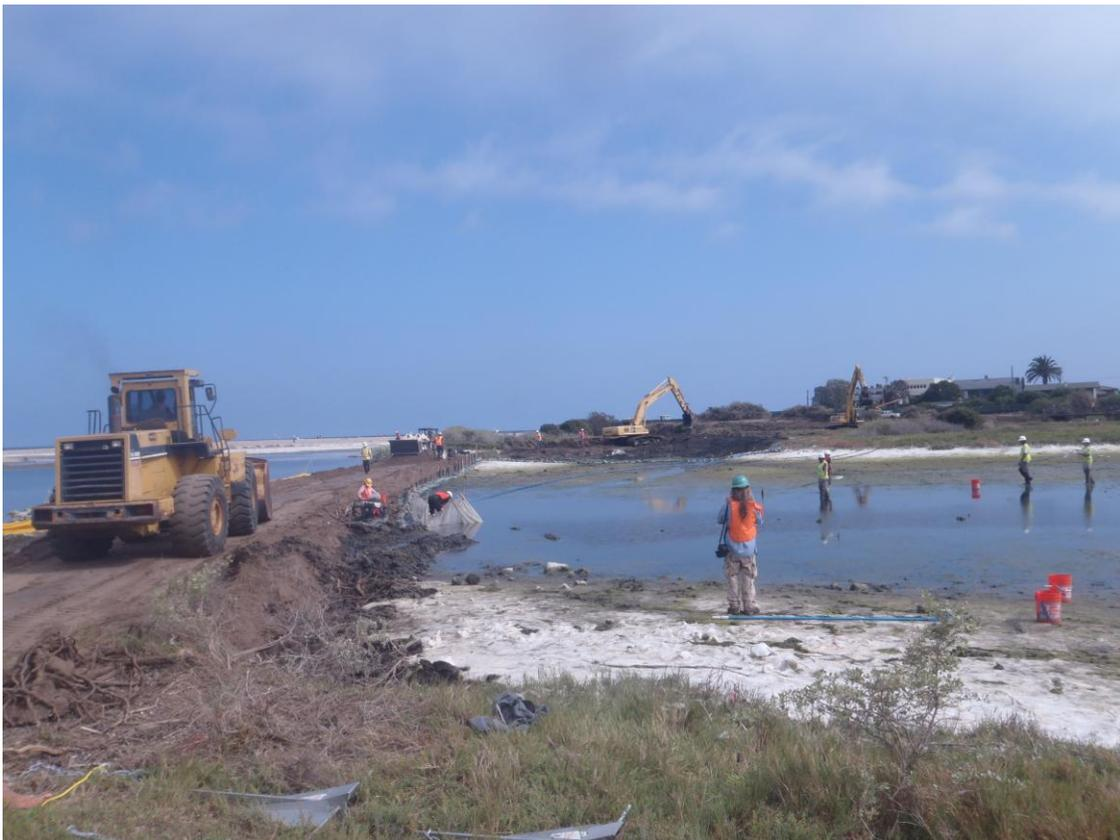
*Photo: Building the earthen dike to block the western channels with fish biologists observing (SMBRF 6/15/2012).*
